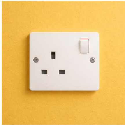
Figure 40 Socket Outlet and Switch with Visual Contrast against Wall
