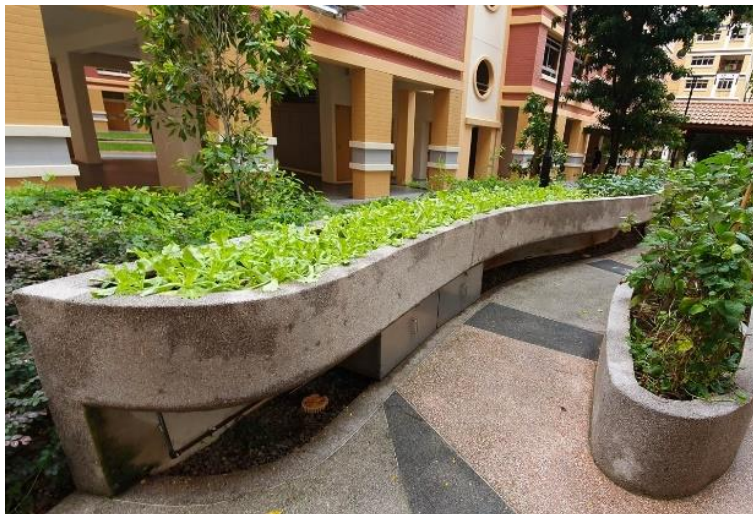
Figure 73 Accessible Planter Boxes
