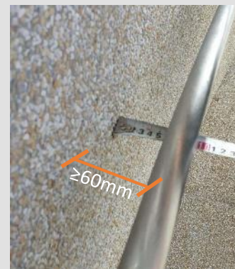
Pebble Wash Wall Surface
