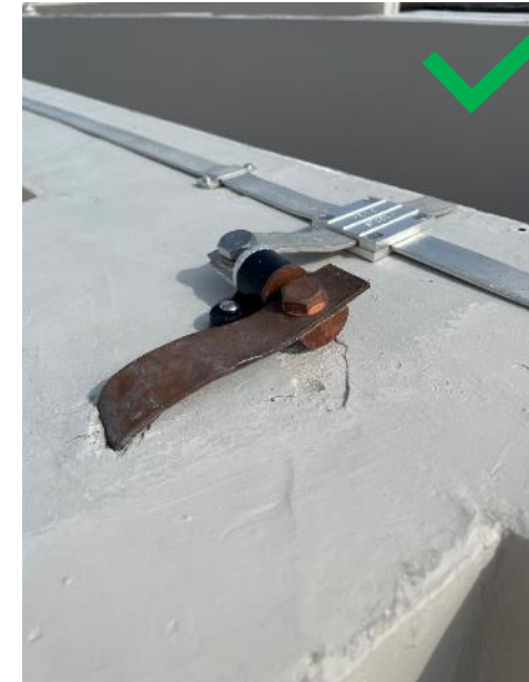
Copper LPS tape embedded in concrete
