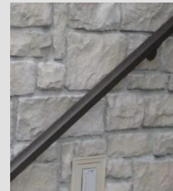
Rough Stone Wall Surface
