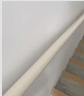
Smooth Plaster Wall Surface
