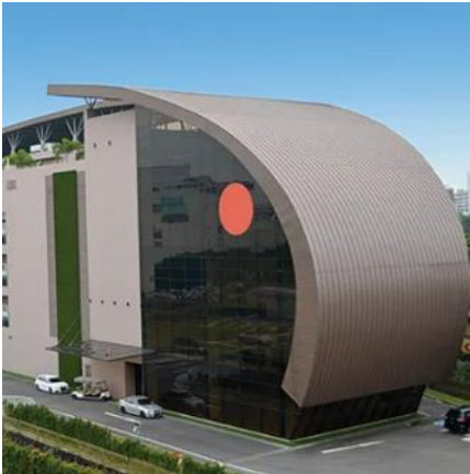
Metal sheet used as both roofing and wall façade
