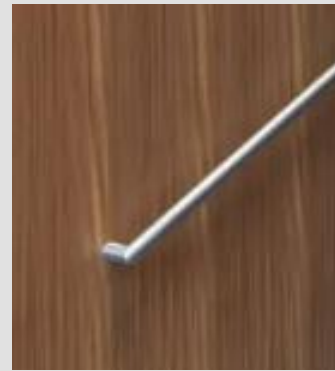
Smooth Timber Wall Surface
