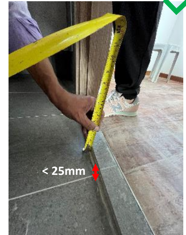
Change in level of floor surface at doorway
