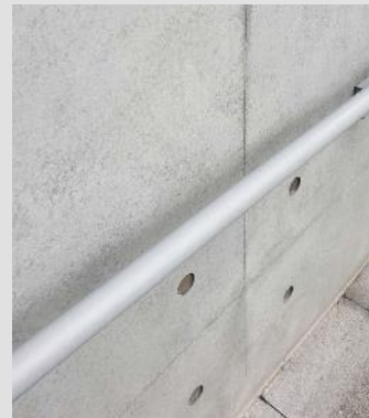
Smooth Concrete Wall Surface
