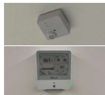
Ceiling sensors and IAQ monitors connected to the Building Management System automatically trigger airflow adjustments to maintain optimal comfort and air quality.
