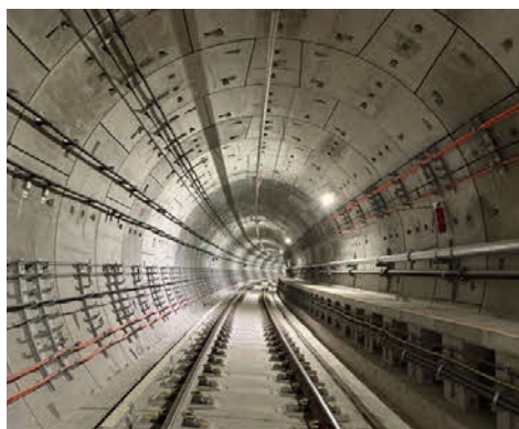
LTA bored tunnels using SFRC segmental tunnel lining.
