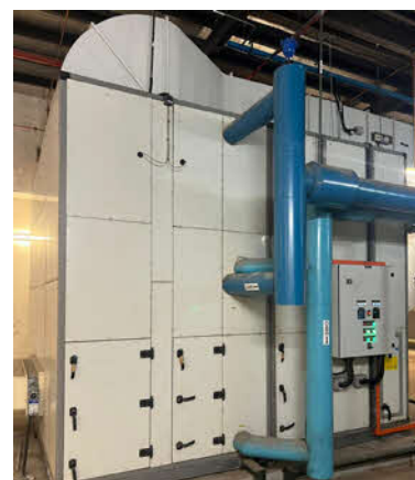
Replaced air handling unit ("AHU") at Blk 27.
