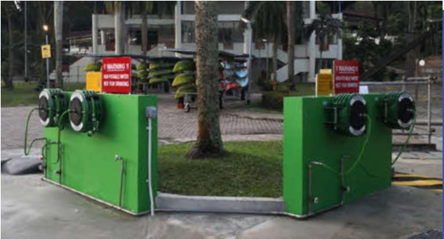
Filtered rainwater is supplied to the washing bay for seacraft and equipment cleaning.
