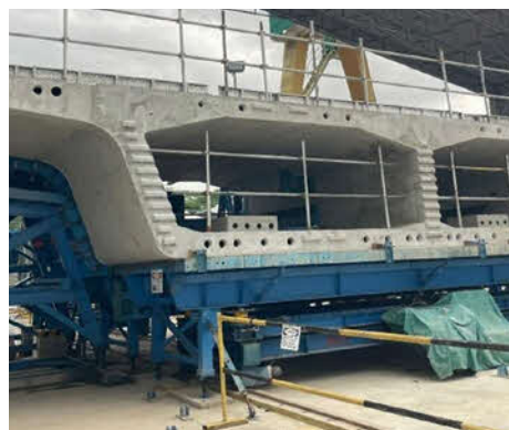
The precast viaduct segment using CMC.
