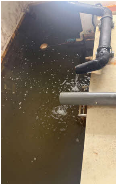
“Reject”water being channelled to NTFGH’s irrigation tank.
