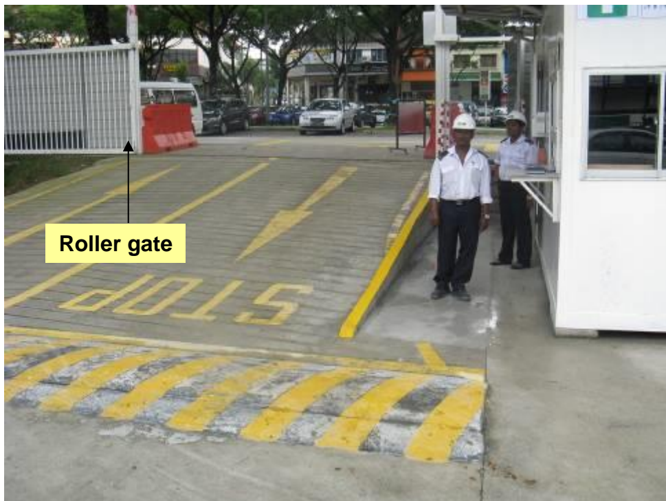
Roller gate at the entrance has an advantage over hinged gate as it eliminates the accidental swinging of gate that can result in hitting man or vehicle
