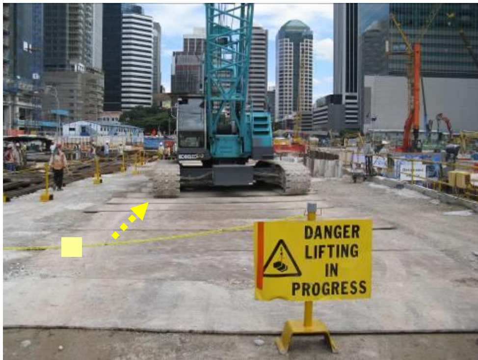
Crane access lined with closely decked steel plates to ensure stability of crane
