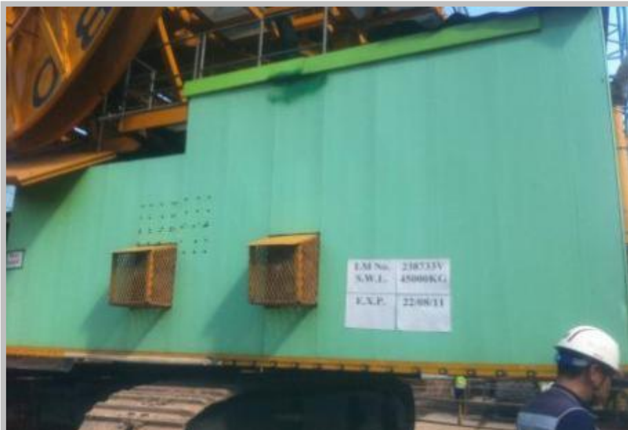
Noise enclosure on D-wall cutter for ventilation fans
