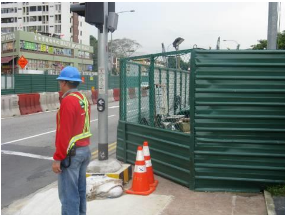
“See through fencing” allows pedestrian to check and ensure vehicles has stopped before crossing at traffic junction
