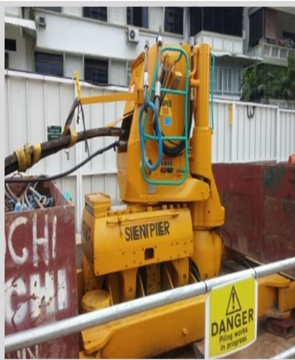
Use of silent-piling machine (for suitable soil conditions)
