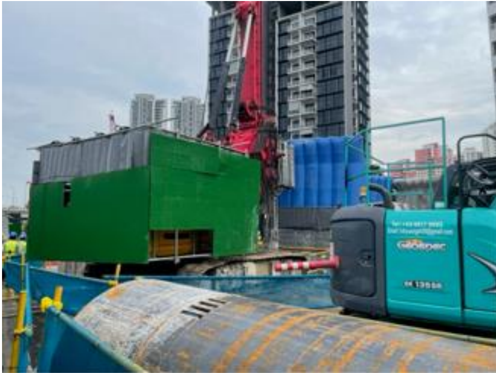
Noise enclosure on boring rigs
