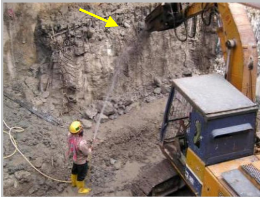
Arresting of dust at source using recycled water
