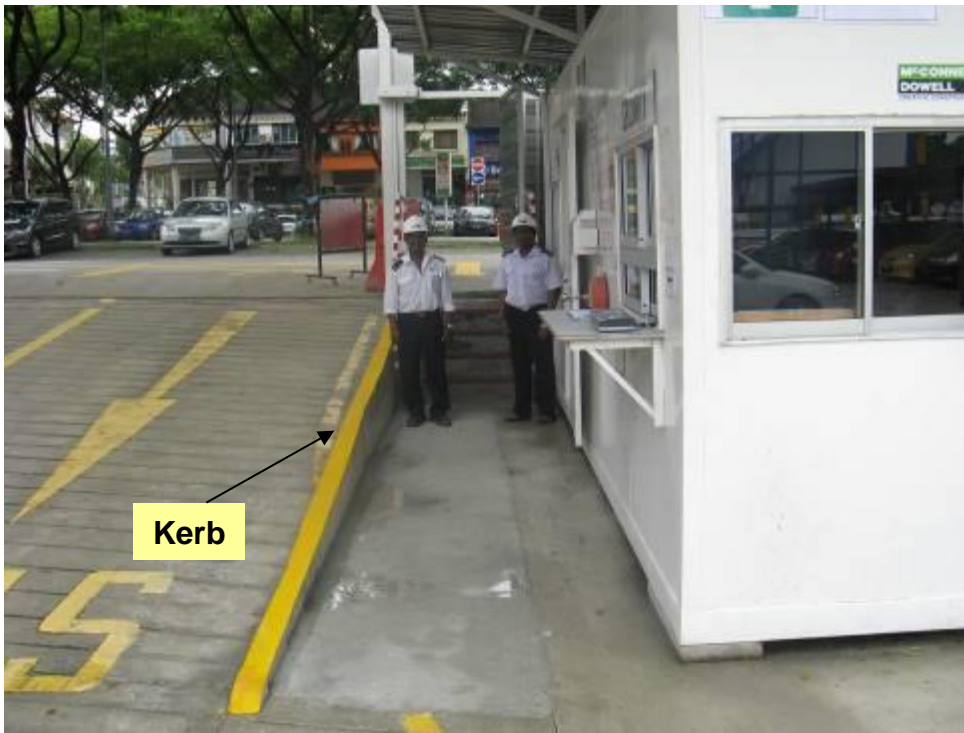
Security pass exchange area separated from vehicle access to prevent vehicles driving too near and injuring workers reporting at the security post
