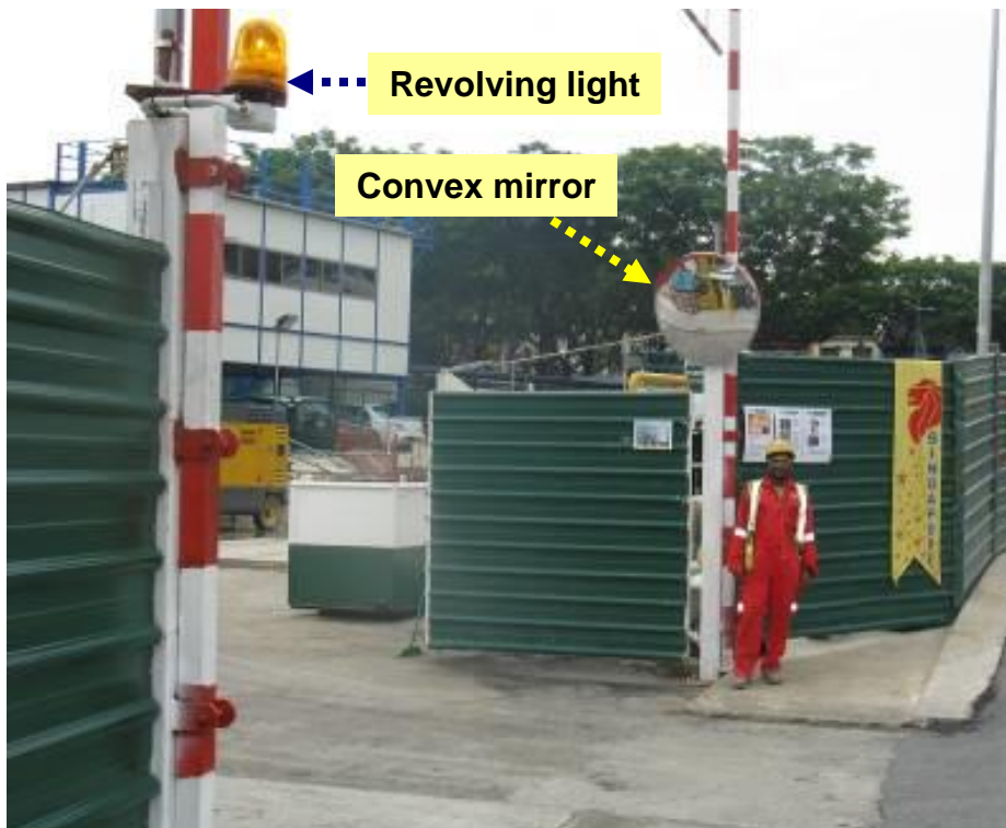
Site entrance equipped with revolving light and convex mirror to enhance pedestrian safety. Full-time banksman deployed to guide vehicles exiting the worksite
