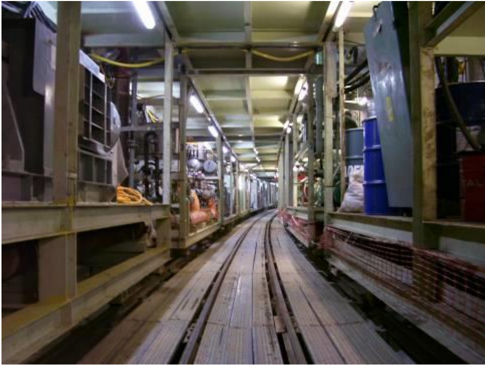
Good illumination and housekeeping maintained underneath TBM Back-up gantry cars
