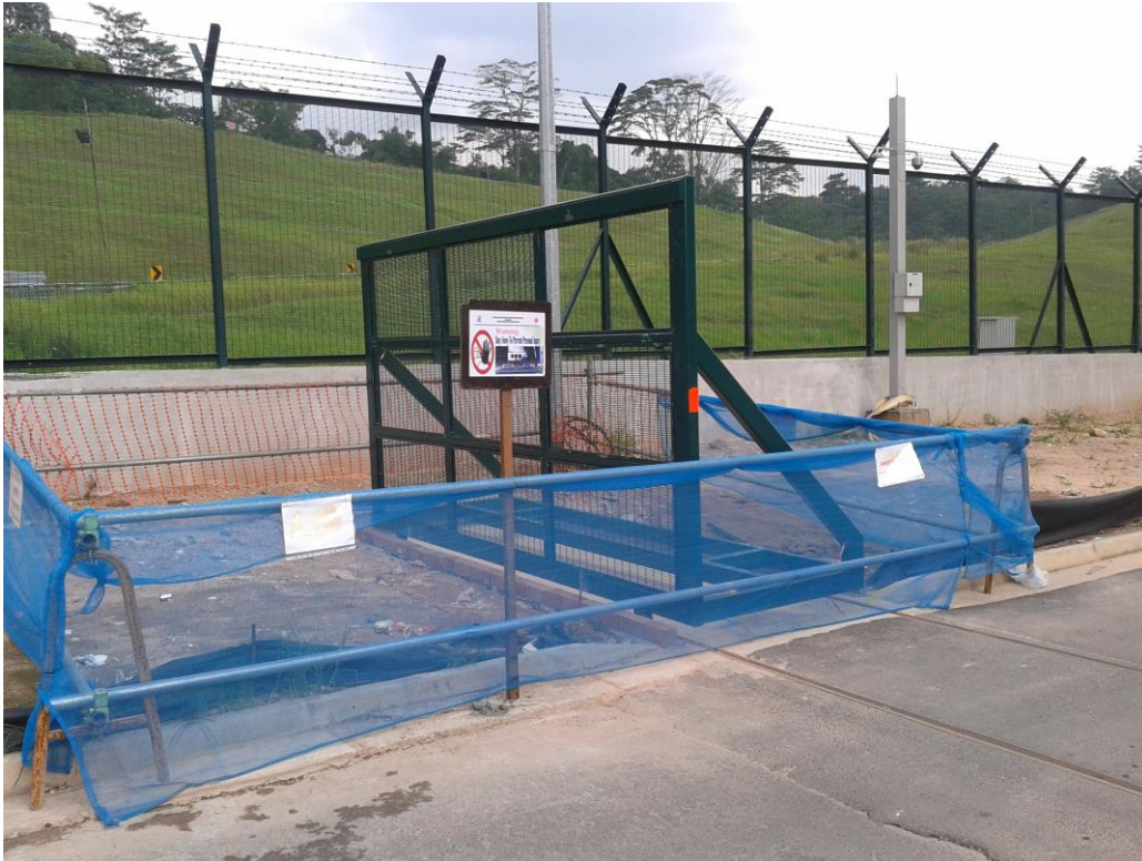
Cordon off work zone around gate installation
