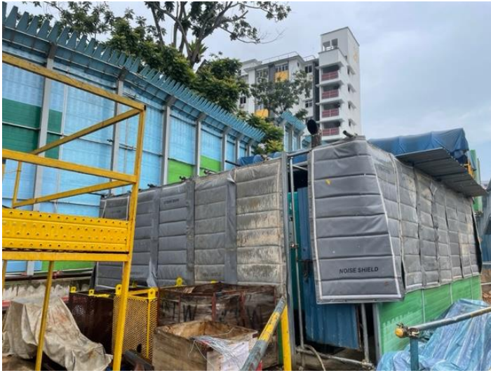
Use of noise shields to house diesel generators
