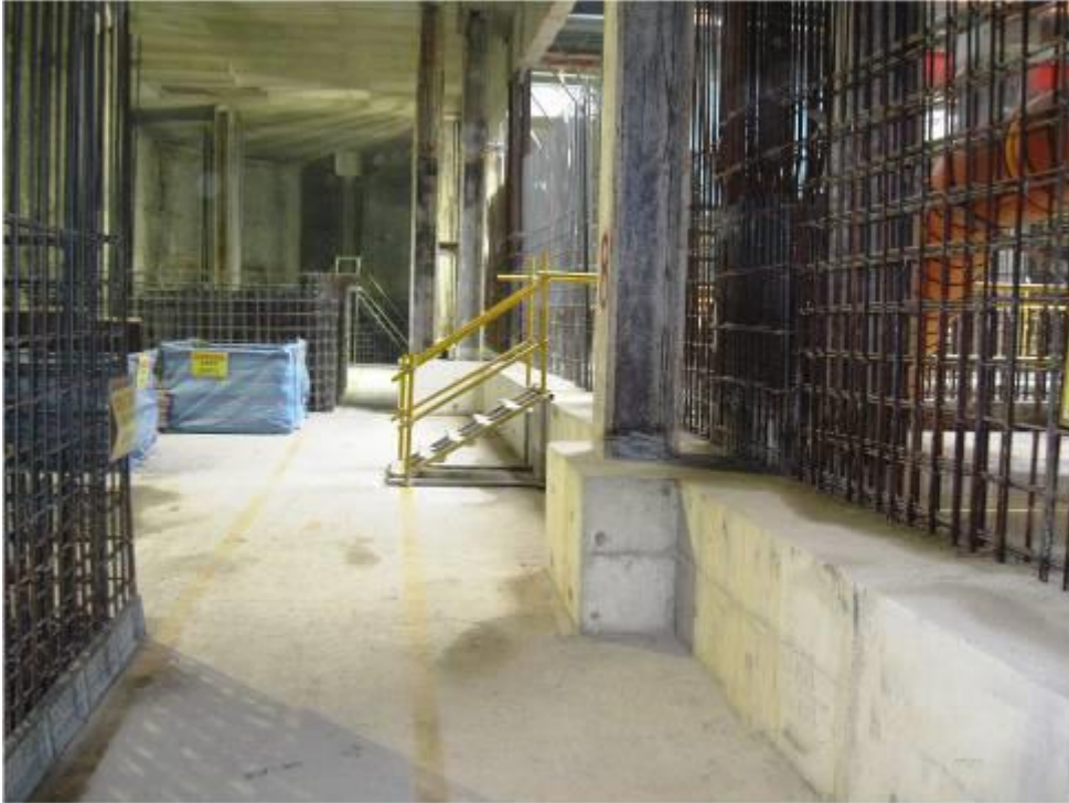
Good housekeeping at worksite with designated areas for storage and walkway
