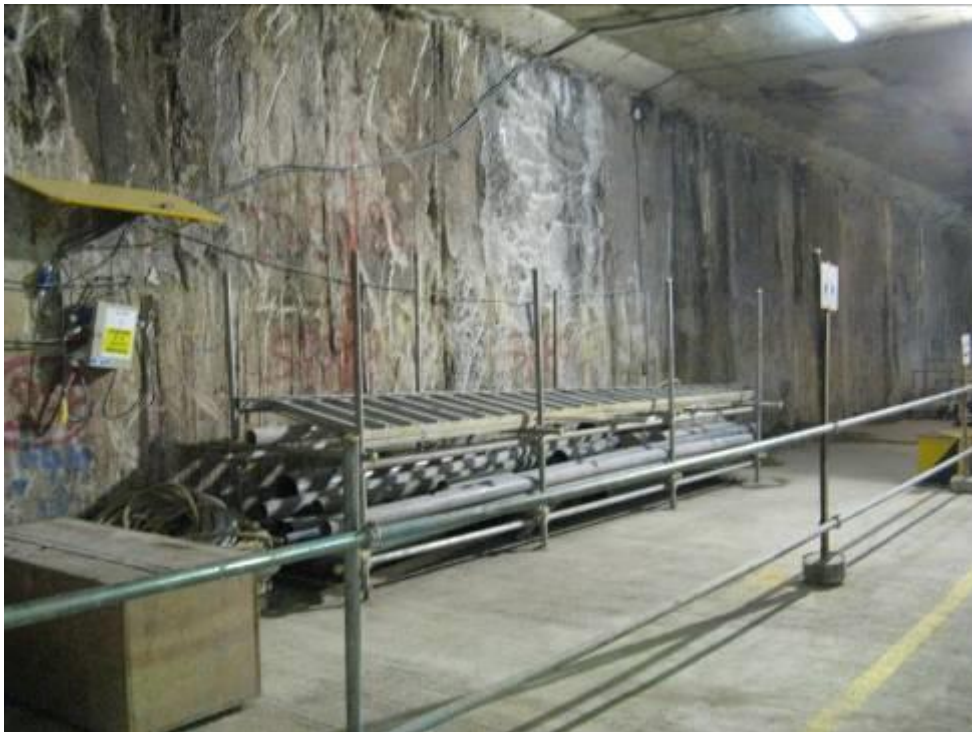
Good housekeeping. Material storage area separate from walkway
