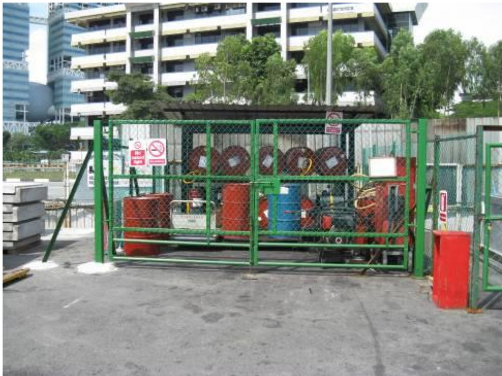
Flammable substance stored at designated storage area with warning signage. Area is locked to prevent unauthorized removal of substance
