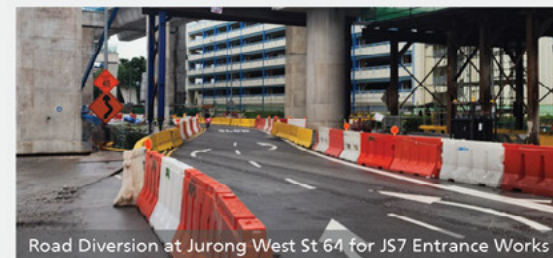
Road Diversion at Jurong West St 64 for JS7 Entrance Works
