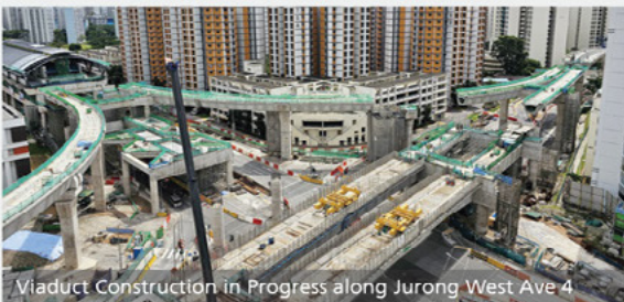
Viaduct Construction in Progress along Jurong West Ave 4
