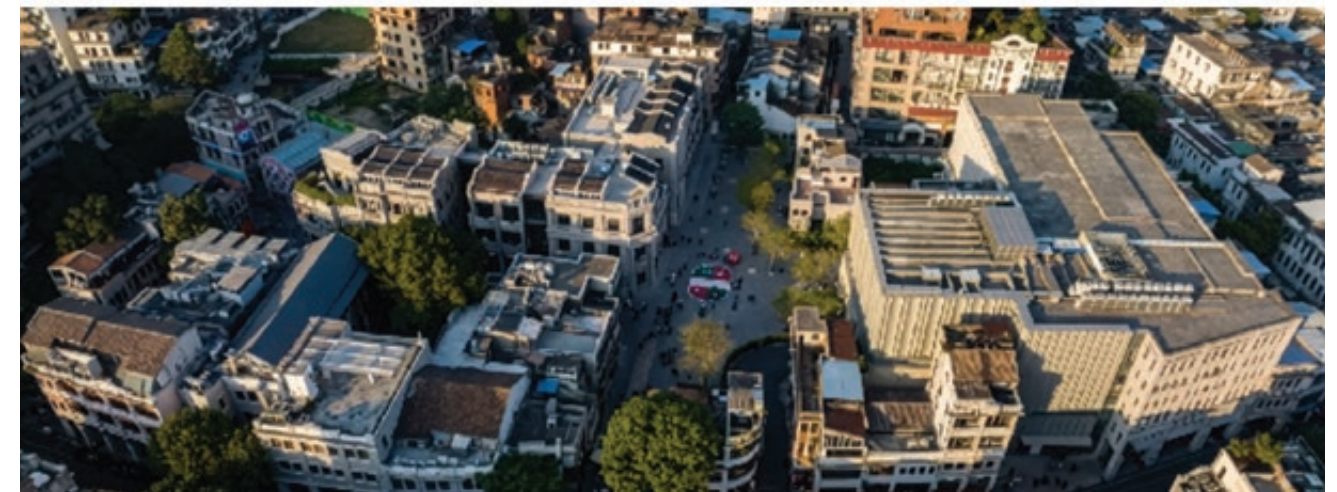
An overview of the Yongqingfang district, before and after restoration. Image: The People's Government of Guangzhou Municipality
