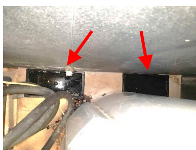
Placement of glue boards along established runways
