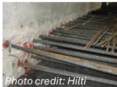
RC slab or beam onto an existing RC wall or column
