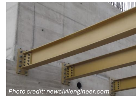
Steel beam onto the RC structure
