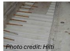
Opening closure / slab enlargement
