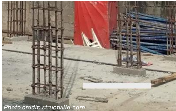
Cast-in reinforcement (Starter bars)
