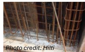
RC slab or beam onto an existing RC wall or column
