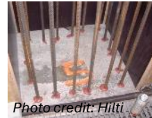
RC column or wall into the foundation
