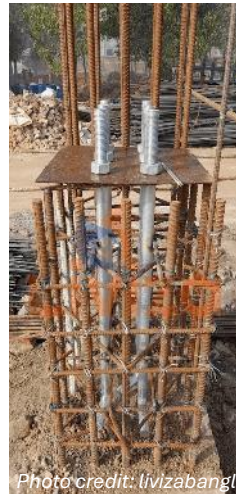
Cast-in anchor bolts
