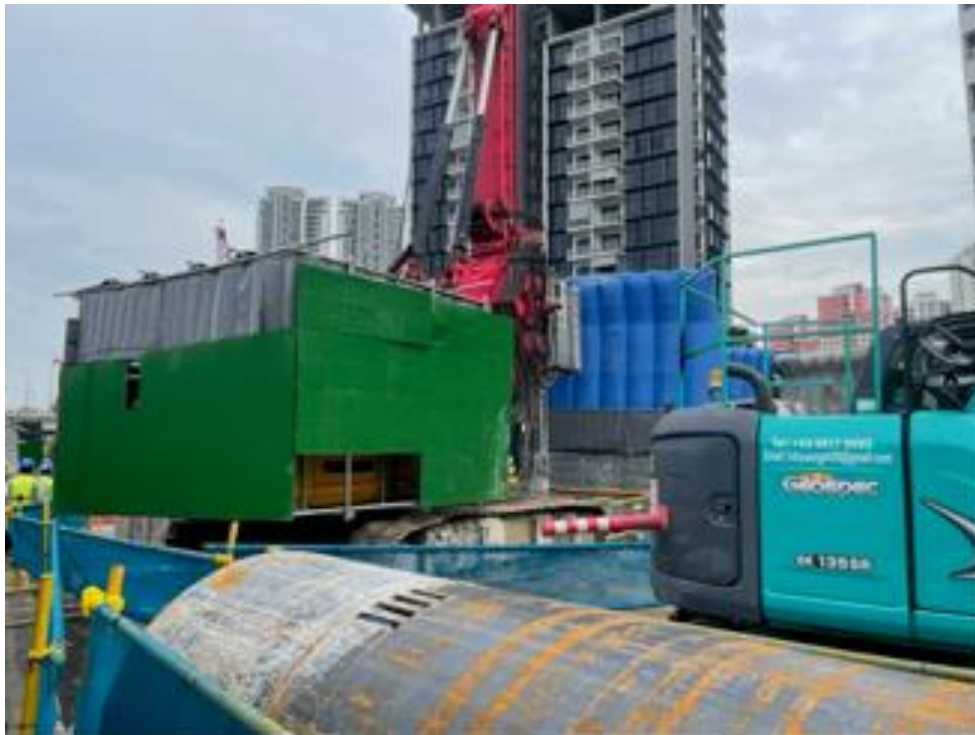
Noise enclosure on boring rigs
