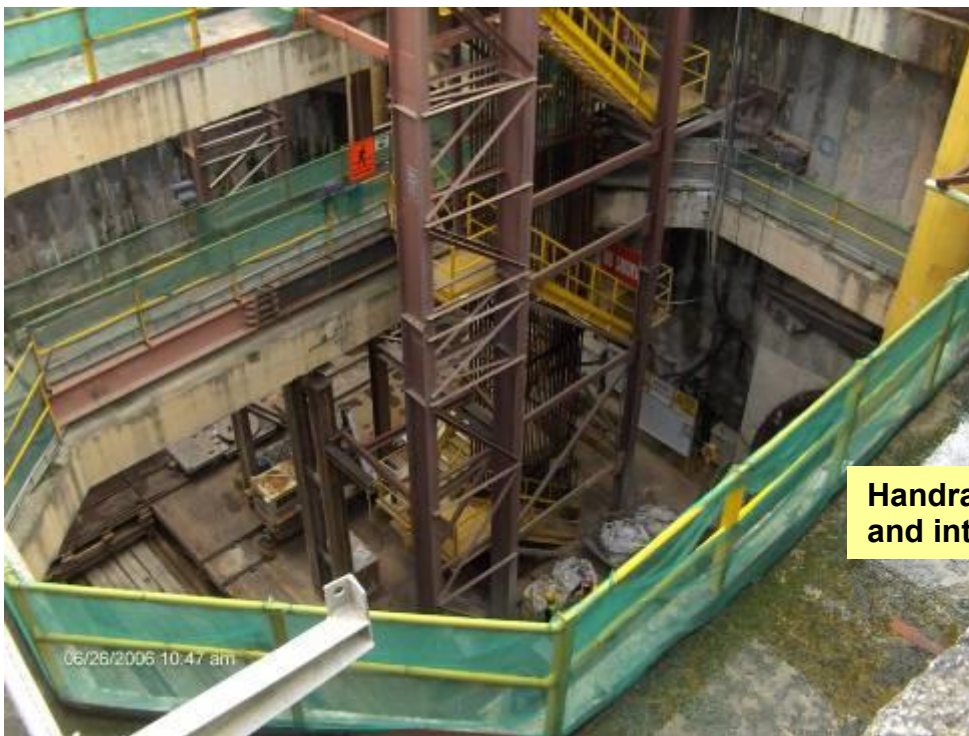
Proper handrails provided at designated site access and walkways. Toe board and netting are added to prevent loose material from falling over
