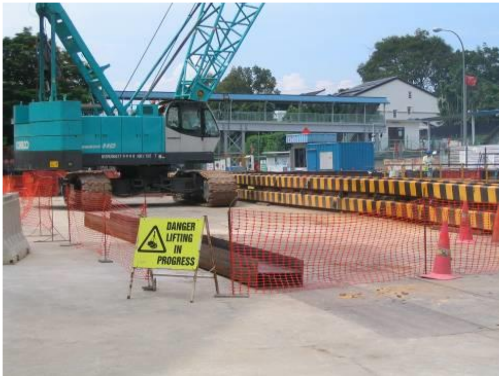
Lifting activity is cordoned off and warning signage is placed to warn personnel against entering the area
