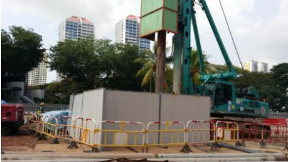
Use of portable noise barriers around noisy works such as bore piling
