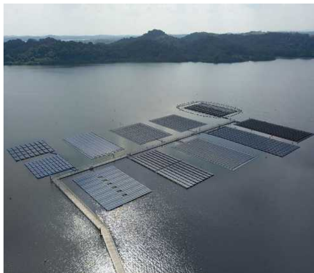
1 MWp floating solar testbed on Tengeh Reservoir.
