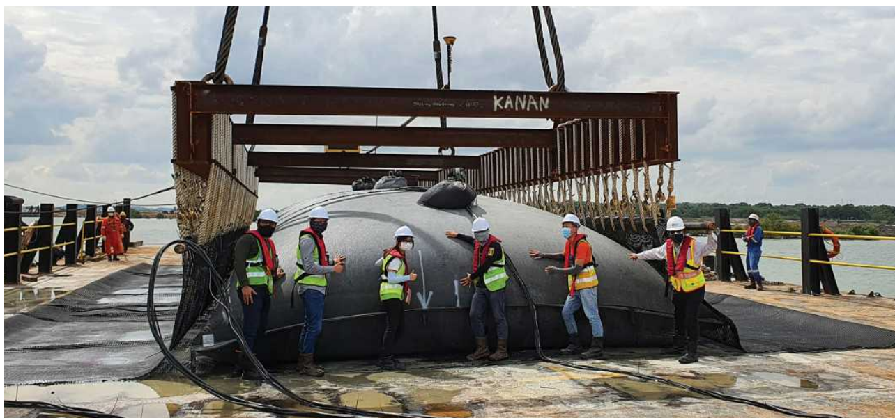
Members of the NUS research team with a full-scale geotextile tube after infilling, secured within the lifting frame specially developed for controlled lifting and underwater installation.
