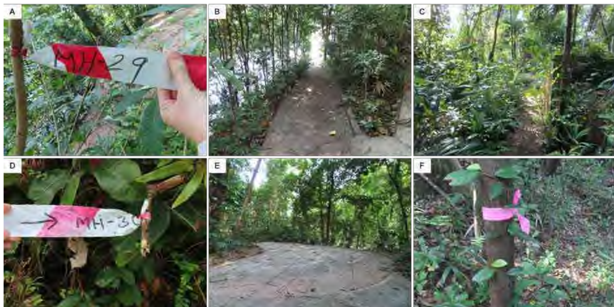
Figure 7-23 Worksites for Manhole MH29 (A–C) and Manhole MH30 (D–F)
