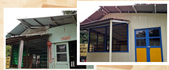
Kampung House Restoration
