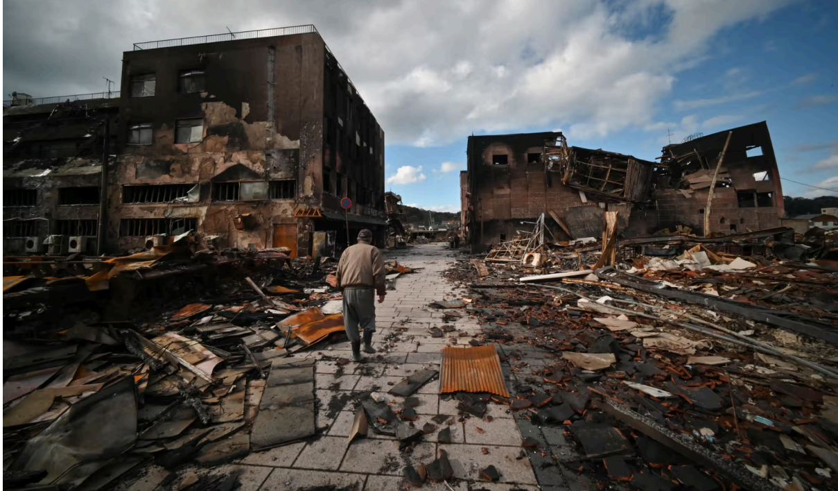
A man walks through the ruins of a shopping district in the city of Wajima, Ishikawa prefecture, Japan after an earthquake. Photograph: AFP/Getty Images
