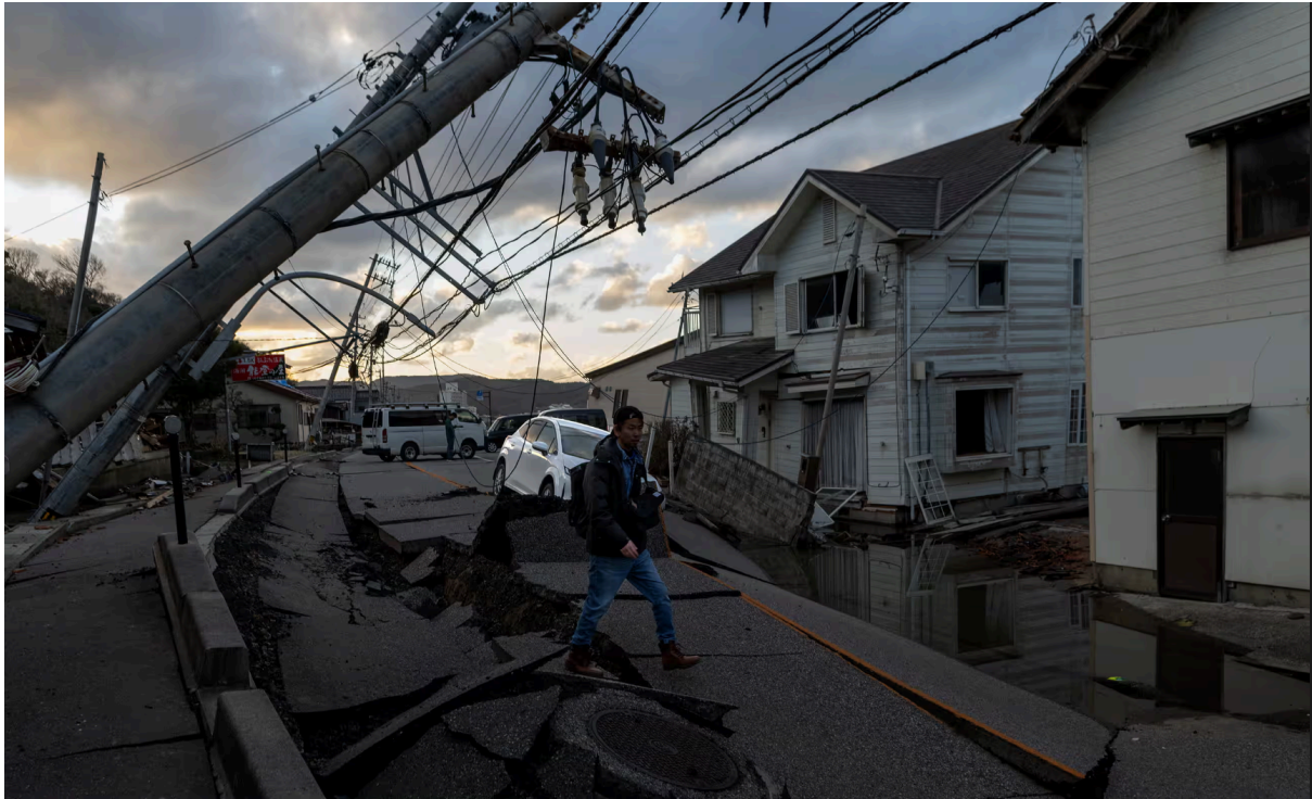
A man walks along a damaged portion of Route 249 amid downed power poles in Wajima, Japan. Photograph: Buddhika Weerasinghe/Getty Images
